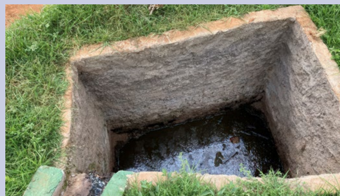
Third pit collecting the digestate used as fertilizer and manually removed with shovels All photos J.Heriniaina, May 2025
