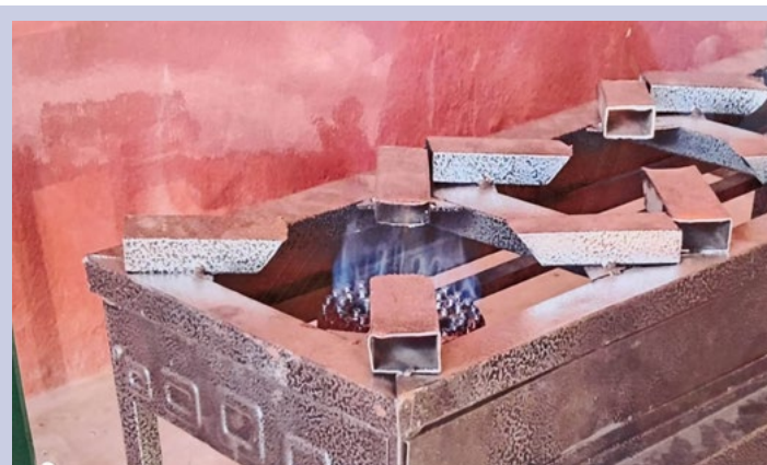
Gas produced being used in the school's kitchen
