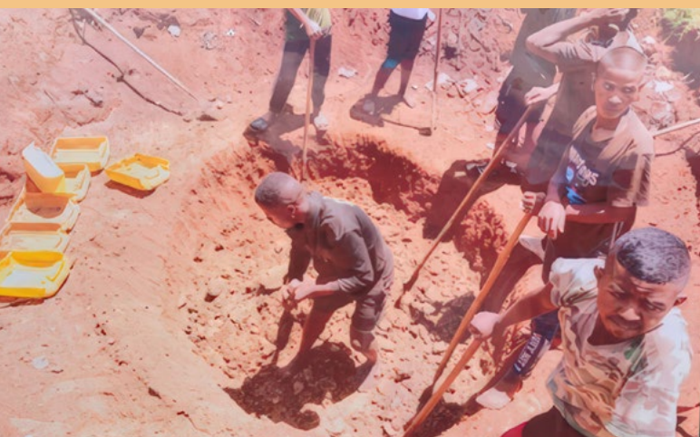
Building a pit for the biodigester J.E. Heriniaina, May 2025
